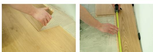
During the installation use a tapping block and a hammer to fit in the boards together along the longer edge. Take care not to spread glue to the tapping block and the top layers of the boards. If the tapping bar and boards are dirty, remove the glue residues using the agent recommended by the glue manufacturer. Glue hardened on the floor surface can cause damage to the walk-on floor layer.
