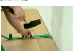
REMOVE ALL EXPANSION WEDGES BEFORE STARTING THE INSTALLATION OF SKIRTING BOARDS. If the floor is to be covered/secured, use breathable material such as regular or corrugated cardboard. Do not cover the floor with plastic materials, e.g. foil. For the floor care and maintenance guide, please visit [www.hardwood-installation.eu](http://www.hardwood-installation.eu). After the skirting boards have been installed, the floor is ready for use.
