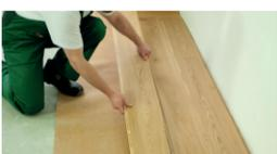
When fitting floorboards using expansion wedges, use an expansion gap of minimum width 7/16" (11mm). An expansion gap should be made along the perimeter of the room and around any other obstructions. Start the installation at the left side of the wall and continue towards the right side.
