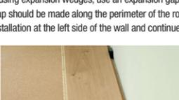
Fit in another board next to the first board. The boards should touch each other along the shorter edge. Begin the second row, starting with the off-cut from the first row. The recommended minimum length for the board starting the next floor row is 12" (300 mm). The recommended offset between the board joints along the shorter edge is 20" (500 mm). Continue laying the floor across the room. Continue laying the floor across the room. Lay the boards at an angle about 30° along the longer edge.
