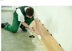
Fit the last board against the wall by tapping it with floor shunting tool. Remember to leave an expansion gap of at least 7/16" (11mm).
