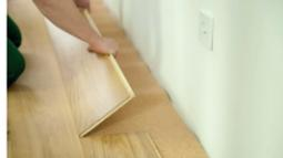
Fit the last board against the wall by tapping it with floor shunting tool. Remember to leave an expansion gap of at least 7/16" (11mm).
