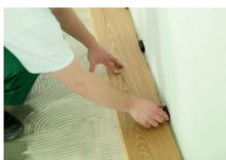
Fit in another board next to the first board. The boards should touch each other along the shorter edge. Begin the second row, starting with the off-cut from the first row. The recommended minimum length for the board starting the next floor row is 12" (300 mm). The recommended offset of connections between the boards along the shorter edge is 20" (500 mm). Continue laying the floor across the room. Lay the boards at an angle about 30° along the longer edge.
