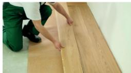
When fitting boards using expansion wedges, use expansion gaps at least 7/16" (11mm) wide. An expansion gap should be made along the perimeter of the room and around any other obstructions. Start the installation at the left side of the wall and continue towards the right side.
