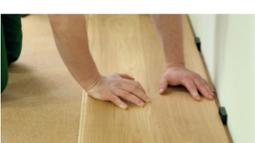
During the installation use a tapping block and a hammer to fit in the boards together along the longer edge. Adjust the tapping block along the entire longer edge of the board and tap it with hammer.
